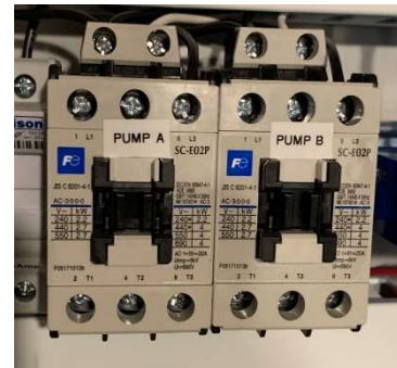
Figure 6: Contactors
